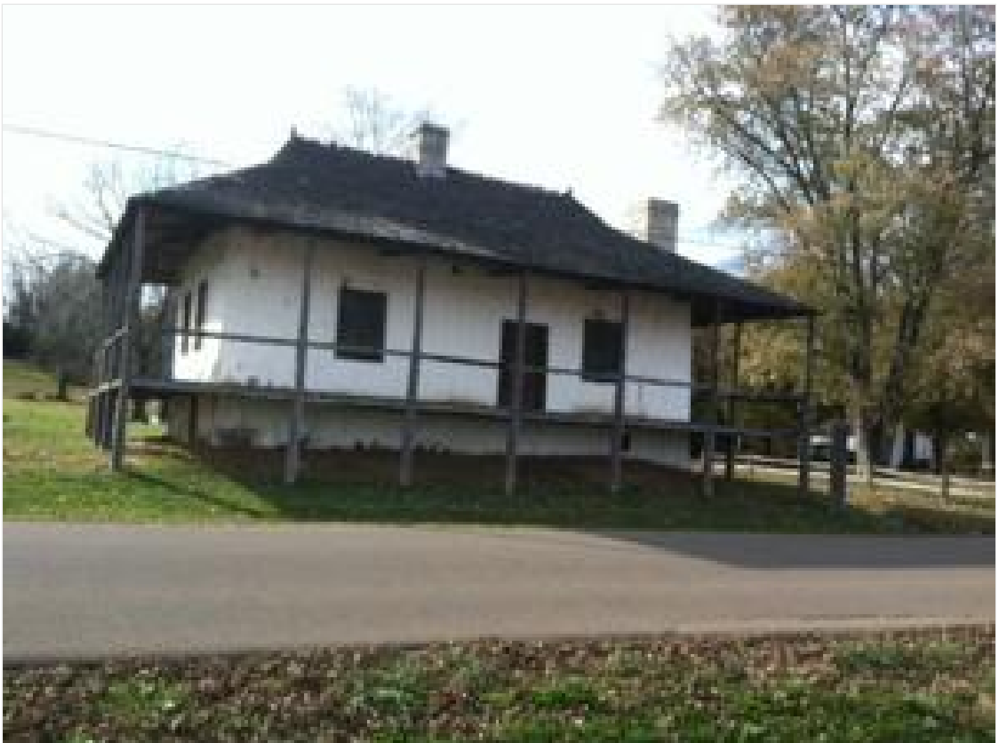
Restoration planned for Bequette-Ribault House in Ste. Genevieve
